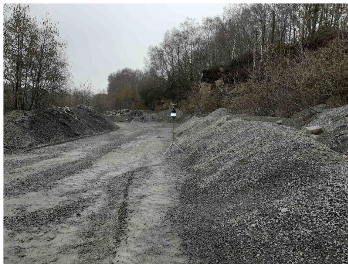
Location D2: north of haul road to Primary Crusher feed hopper (located in a side area not currently subject to any haulage movements)
